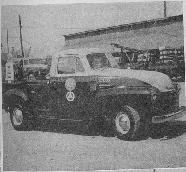
Emergency Power Supply and Equipment Transporta- tion, for Civil Defense.
