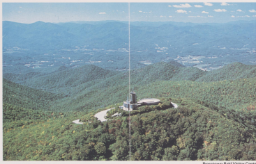
Brantstown Bald Visitor Center
