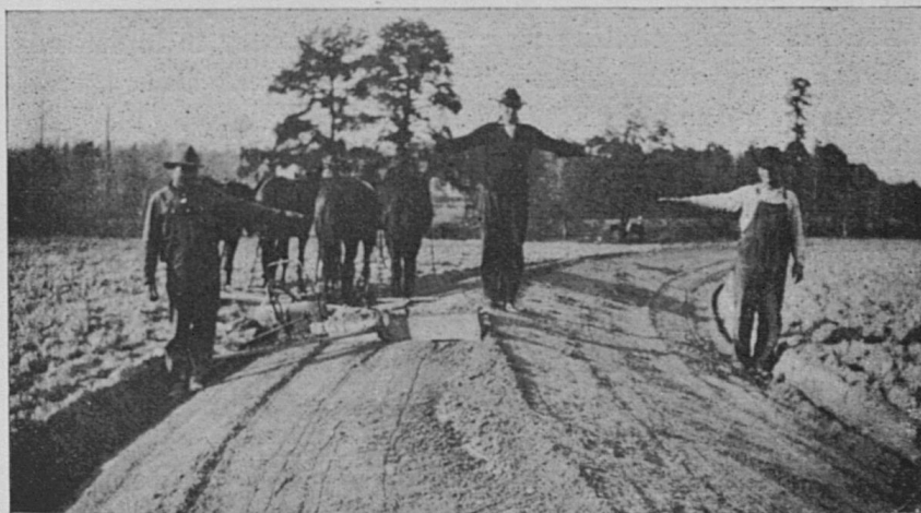
Fig. 9. Finishing a broad-base terrace.
