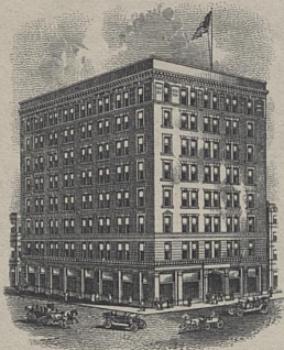
TRUST COMPANY BUILDING.
