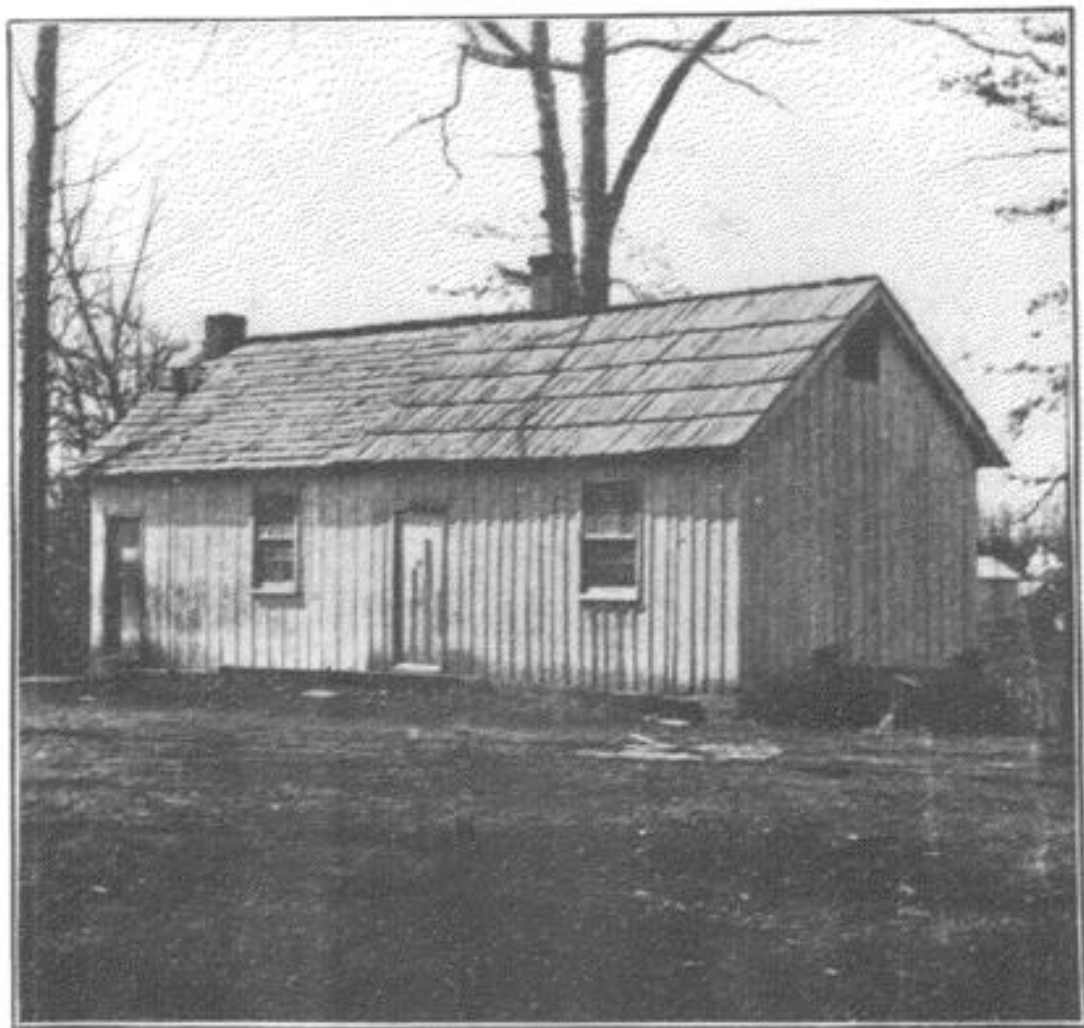
No. 2—SECOND OF THE COLLEGE BUILDINGS.
