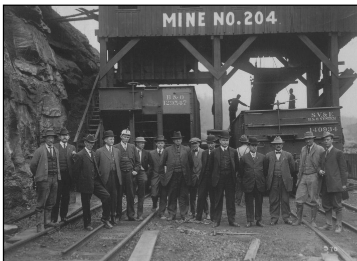
Photo: Big Sandy Operators stand at a coal mine tippie, used to load coal onto railcars on March 26, 1914. Jenkins, Kentucky Photographic Collection, University of Kentucky Special Collections .
