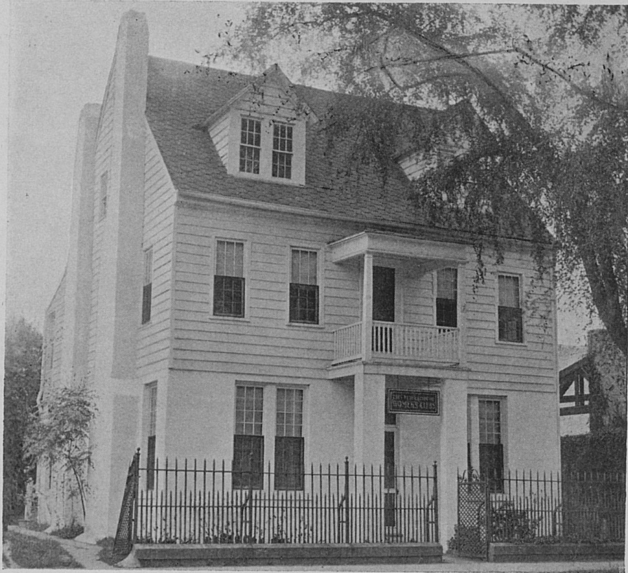
WOMEN'S CLUB BUILDING, SHOWING EARLY ARCHITECTURAL TREND IN AUGUSTA
