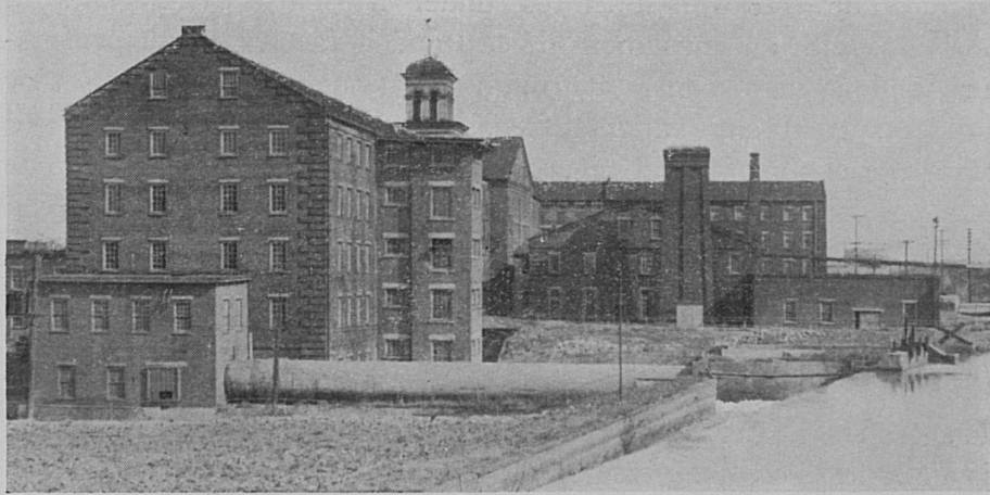
AUGUSTA FACTORY ON THE CANAL BANK
