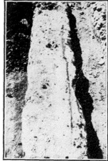
This old stone sill, which formed a part of the foundation of the old Lexington & Ohio track, was unearthed at Lexington, Ky.
