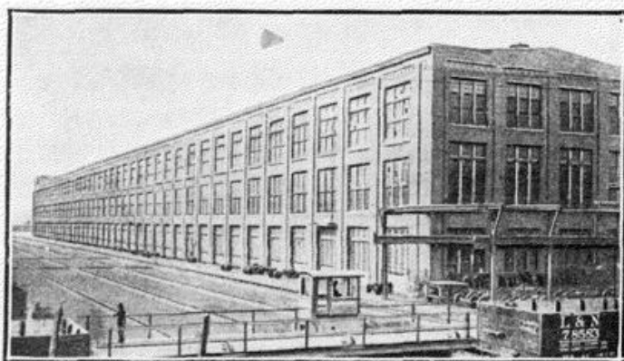
View of a Portion of One of the Machine Shop Buildings of the L. & N., South Louisville, Ky.
