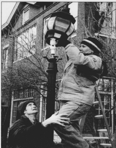
PHOTOS BY ELLIOTT HESS/STAFF Grounds crew workers Bedia Collins, right and Don Dugal change an energy-efficient fluorescent light bulb in the front yard of Maxwell Place on Jan. 25.
