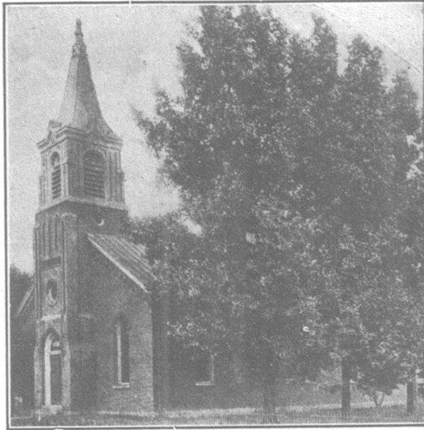
PRESBYTERIAN CHURCH Erected in 1827
