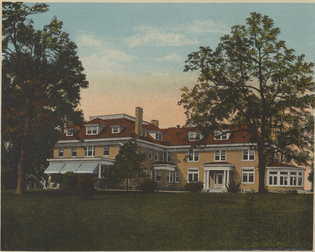
FRONT VIEW, SHAFFER MANSION.
