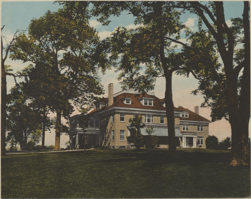
SIDE VIEW, SHAFFER MANSION.
