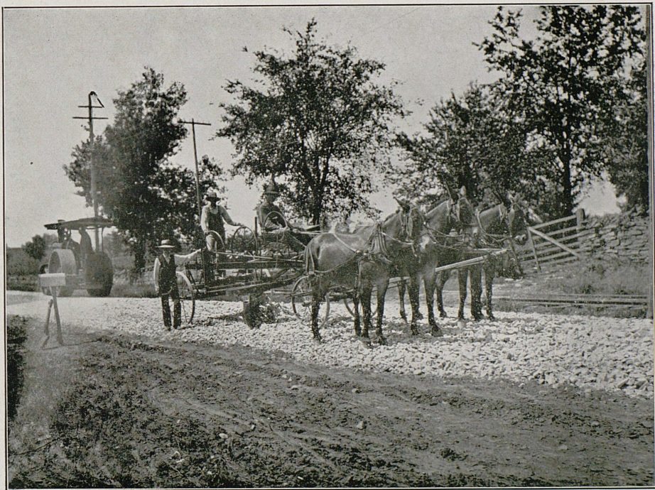
Grading and Rolling a Road.
