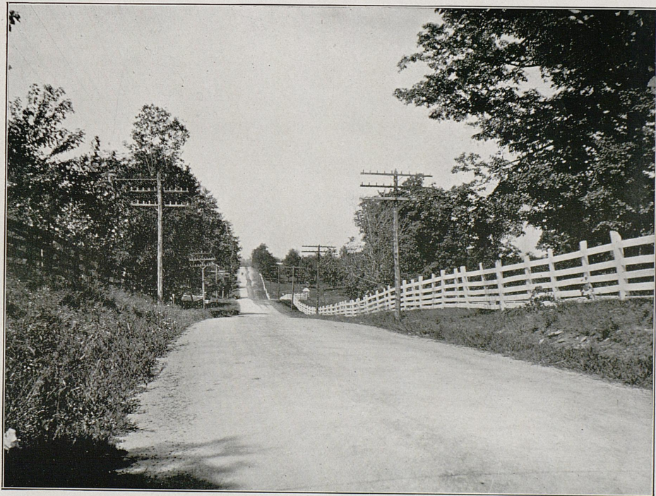
Winchester Road at Patchen Wilkes Stock Farm.
