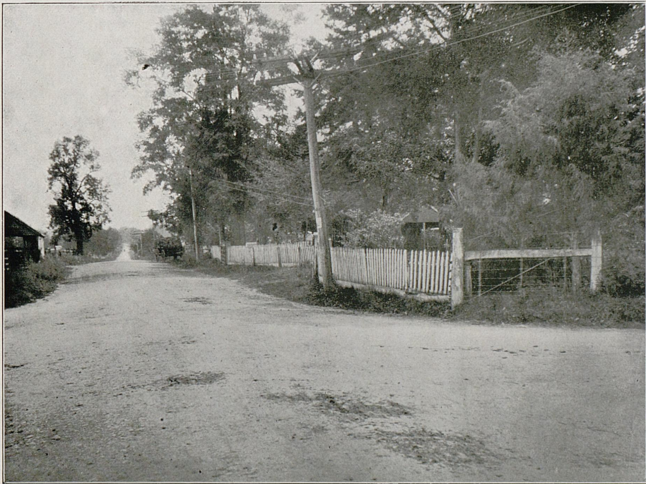
Intersection of Newtown and Iron Works Road.
