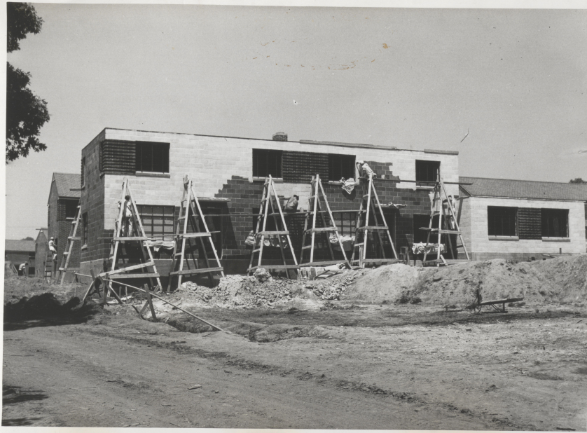
54 RA682-D-FINISHING TOUCHES TO A MODERN DESIGN. Flat roofs and vari-colored paint will beautify homes for residents of Greenbelt who want the modern touch in architecture. The houses shown here are of cinder-block construction. Others are of brick. In all cases, however, foundations are of poured concrete, and in the cinder-block, modern houses the roofs also are of poured reinforced concrete topped with high grade roofing materials. Rows of boxes masquerading as homes won't be found here. Greenbelt homes are designed to combine beauty with practicability. Within the next few weeks shrubs will be planted to give a park like appearance to the super-blocks in which the groups of houses are spaced. From the houses in the picture residents will look out on the fields and hills of the greenbelt, that broad girdle of farms, parks and gardens which surrounds the town. Not only will there be professional farmers to work the farms but those residents who wish it may have allotment gardens here in which to raise crops for home use in spare time. Picnic grounds and a beautiful artificial lake will complete the recreational value of the greenbelt region from which the town gets its name. (Resettlement Administration Photo)
