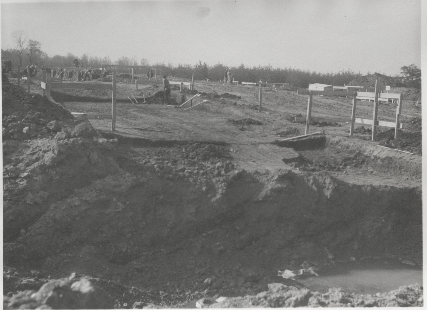
3. MACHINE EXCAVATION COMPLETE - START OF EXCAVATION FOR FOOTING
