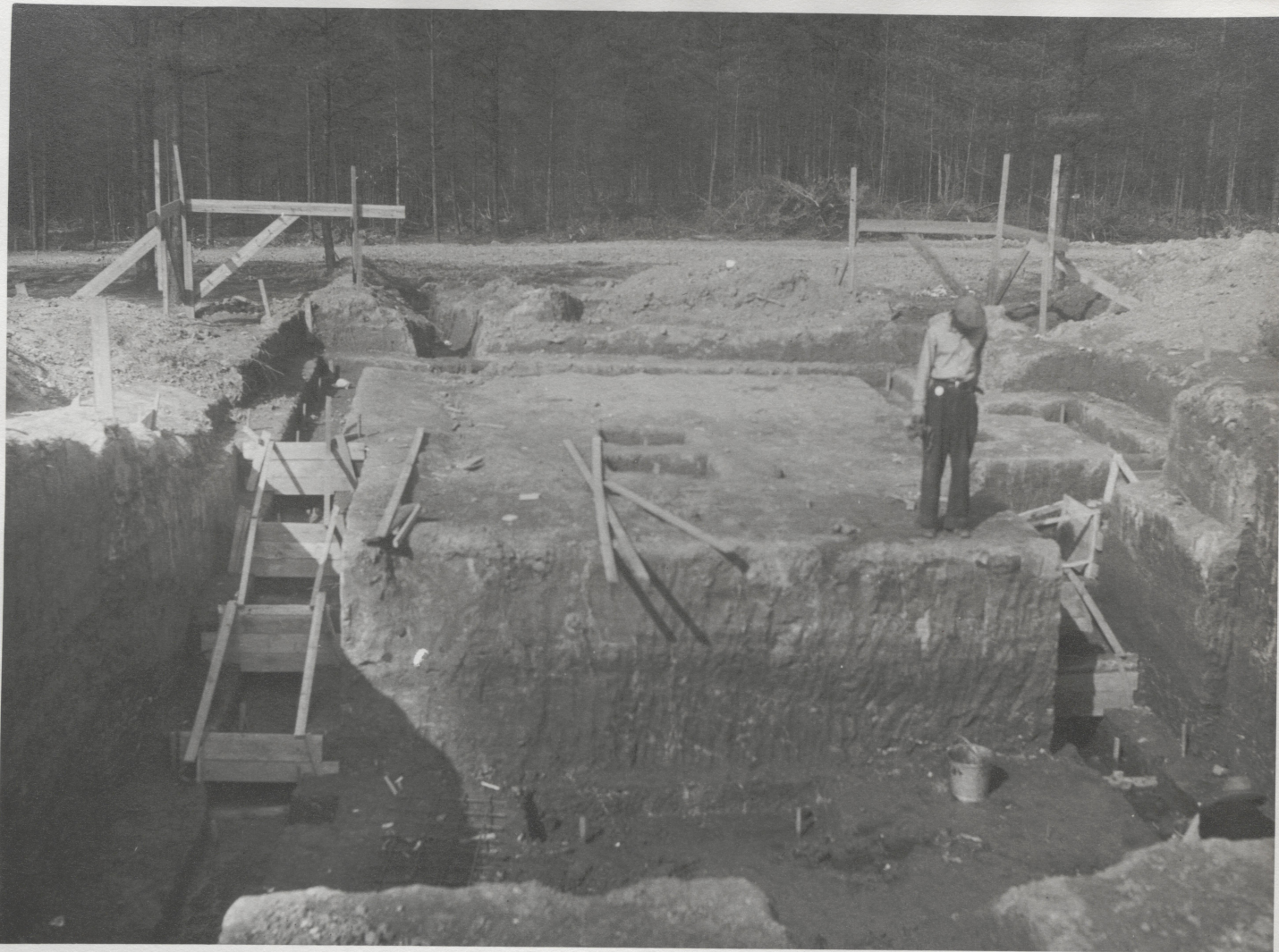
4. FOOTING EXCAVATION COMPLETE
