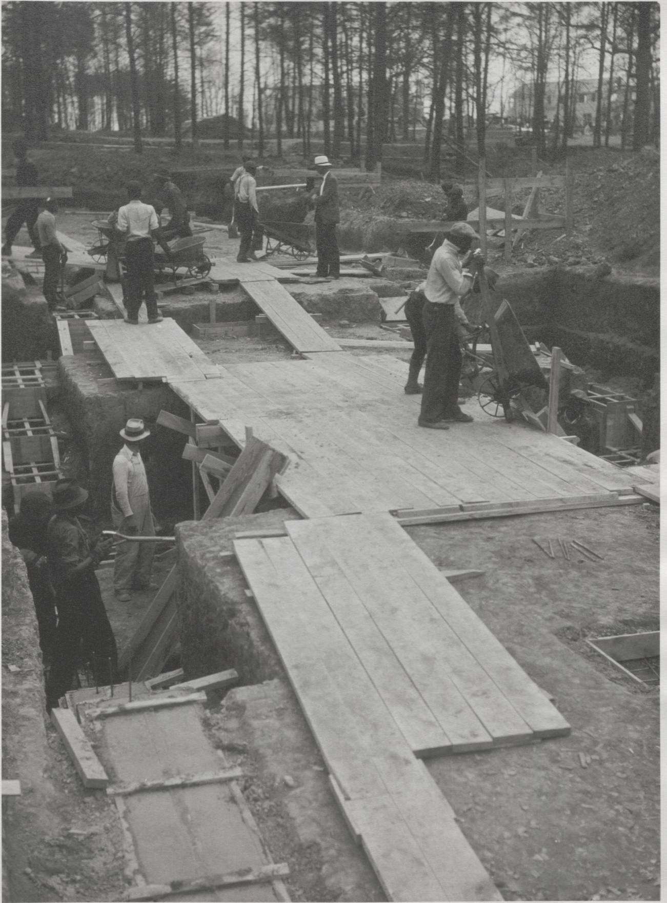
5. POURING CONCRETE IN WALL FOOTINGS
