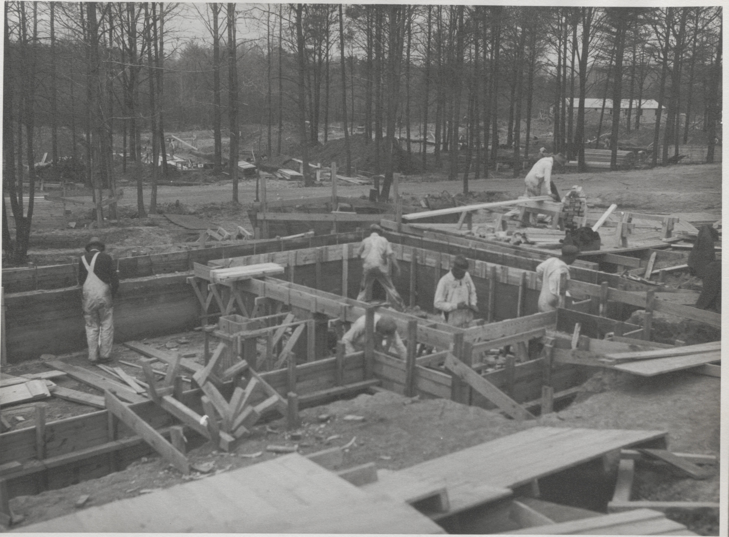
7. WALL FORMS AND WALL REINFORCING STARTED
