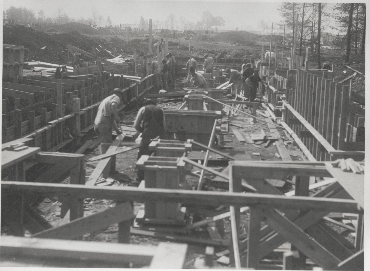
8. WALL FORMS COMPLETE
