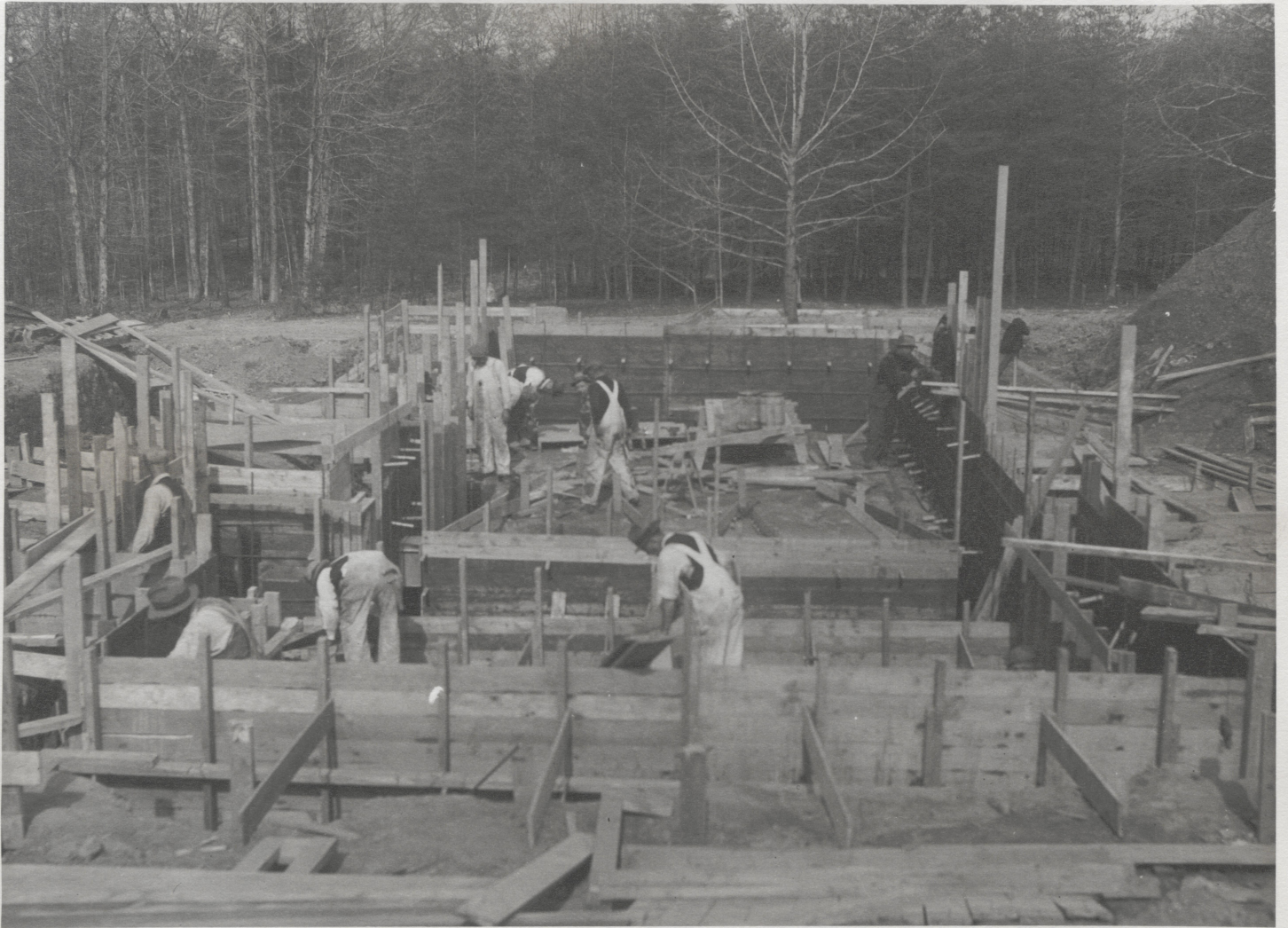
10. WALL FORMS STRIPPED - 1st FLOOR BEAM FORMS BEING FRAMED
