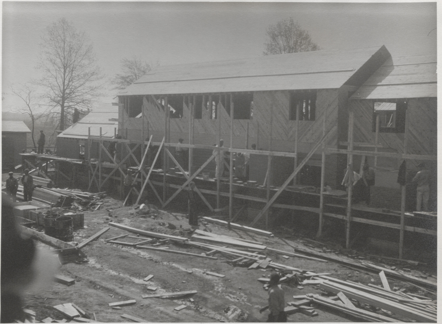
18. BRICK WORK STARTED - SHEATHING NEARLY COMPLETE
