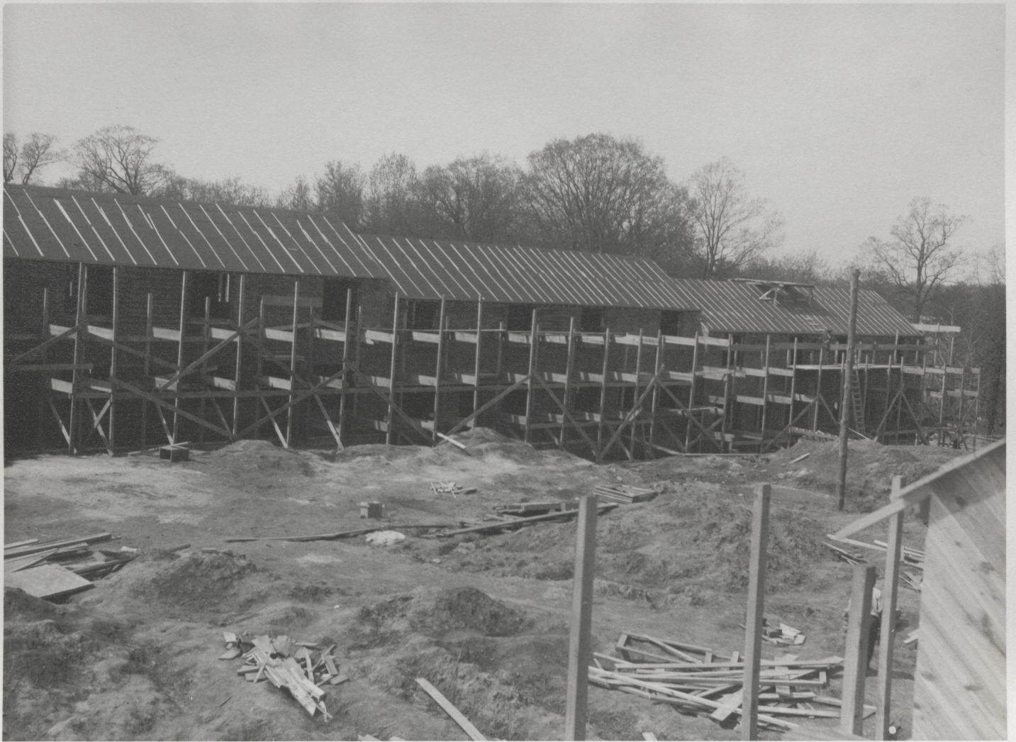
19. BRICK WORK COMPLETE - ROOF PAPERED
