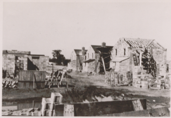
HOUSES UNDER CONSTRUCTION ILLUS. NO. 25
