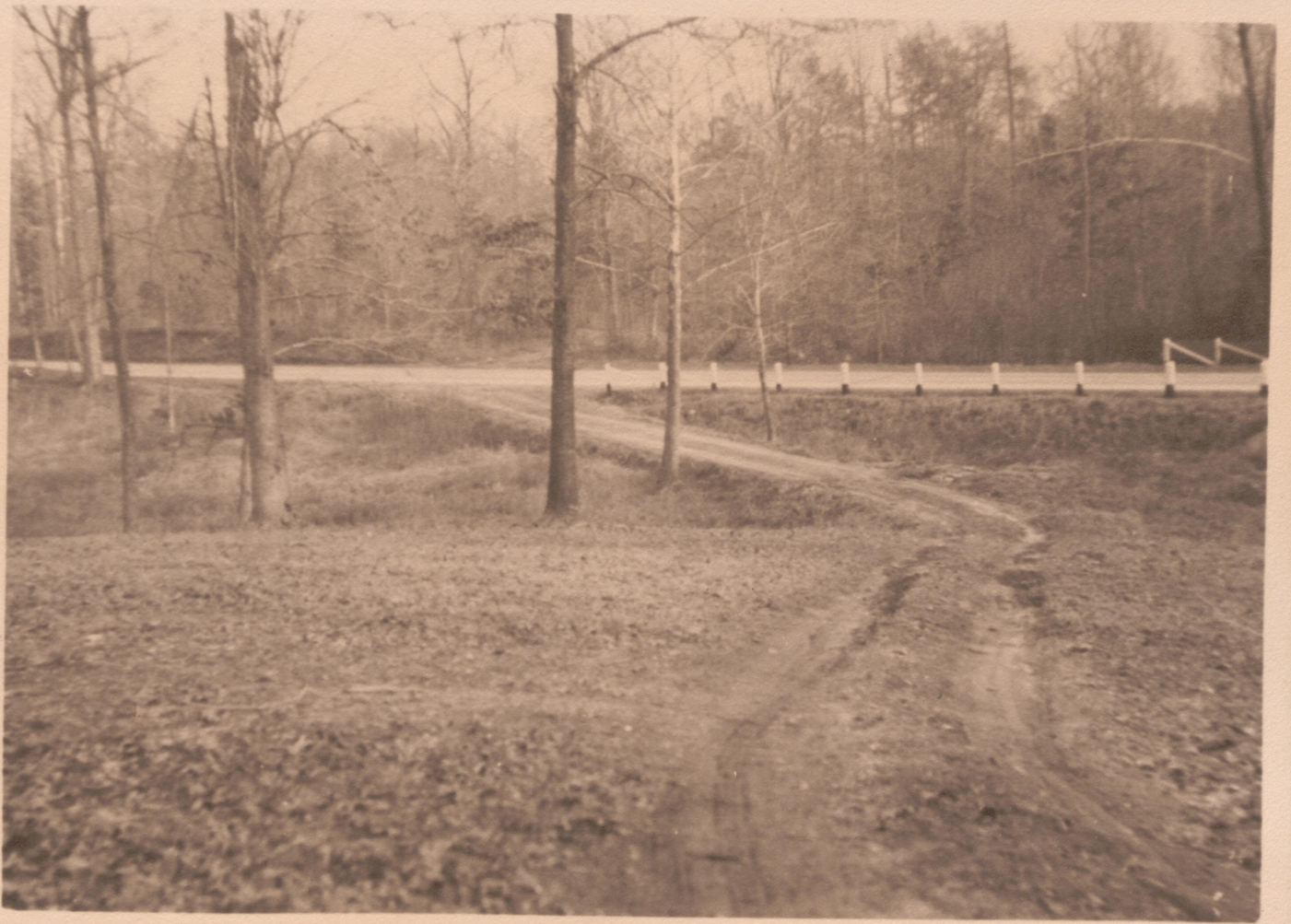
NO. 1. U. S. ROUTE 1 AT SOUTH BOUNDARY
