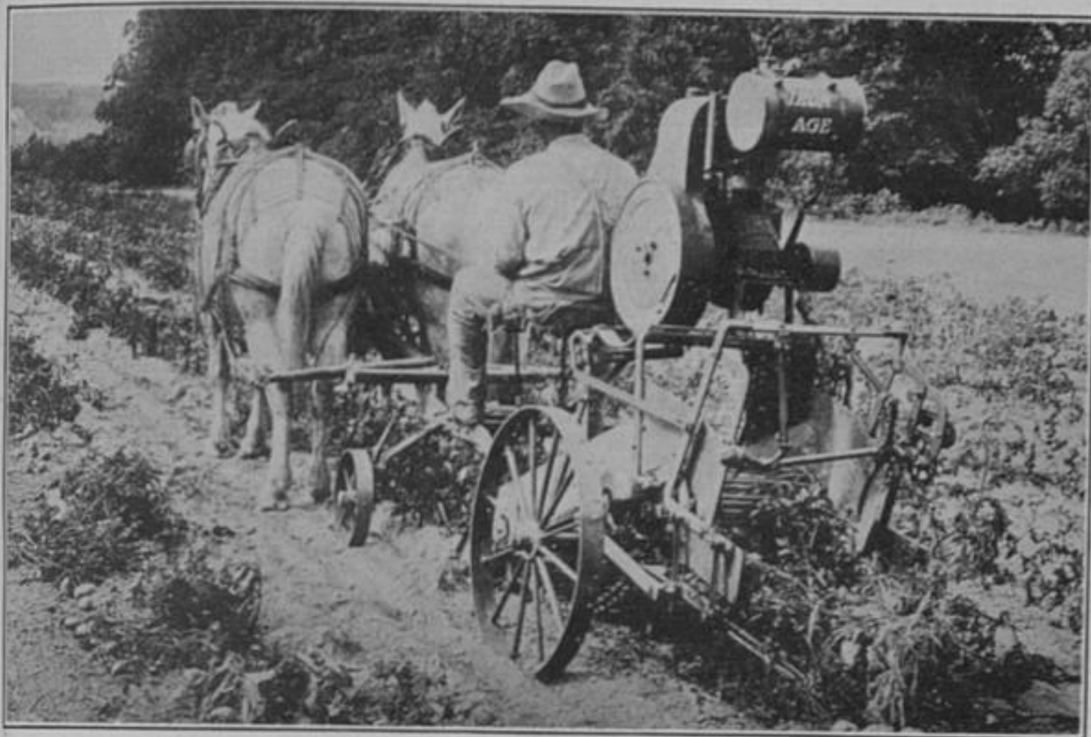
Elevator type of potato digger. The gasoline engine mounted on the digger takes the place of extra horses.
