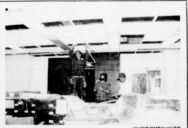
Three employees from the National Ace Construction Company install the new sprinkler system in the Patterson Office Tower.
