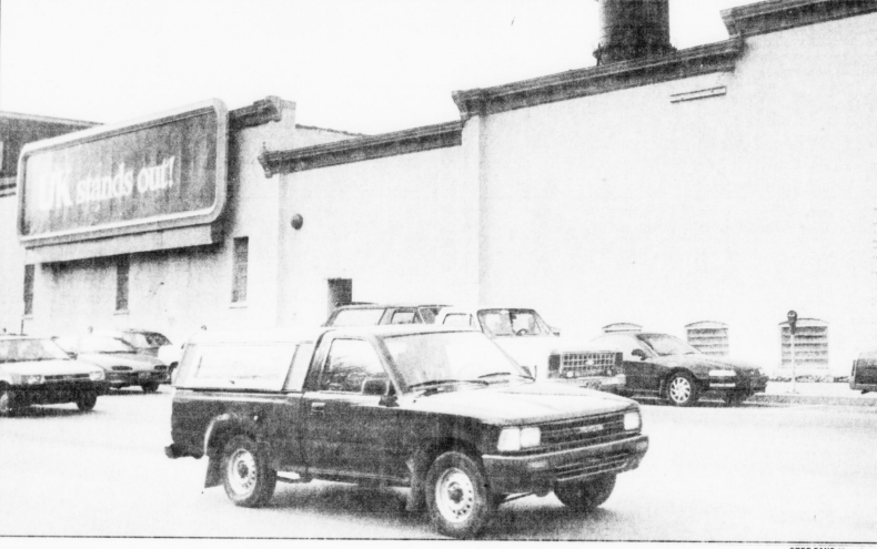
COMING DOWN UK's new parking structure, scheduled to be completed next year, will replace the American Building at Euclid Avenue and Limestone Street.
