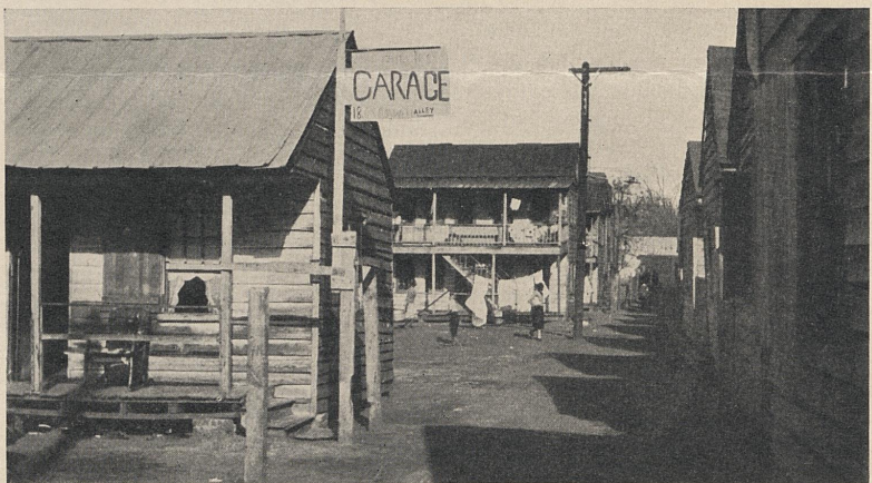
This view of the slum dwellings which formerly occupied the site of Robert Mills Manor in Charleston, S. C., was taken from the same spot as the picture on the opposite page, which shows the project nearing completion.
