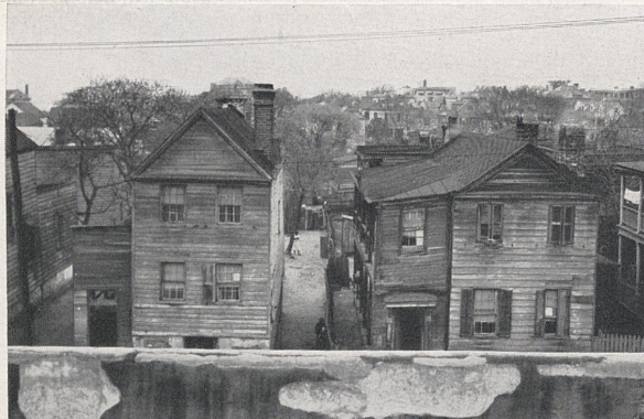
The site of Robert Mills Manor, Charleston, S. C., before demolition.
