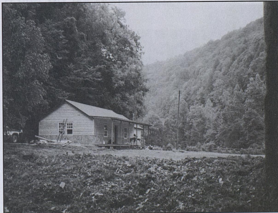
The newly renovated Hurricane Workshop - The Livery
