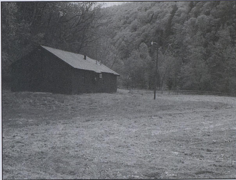
The Wendover Hurricane Workshop before renovations
