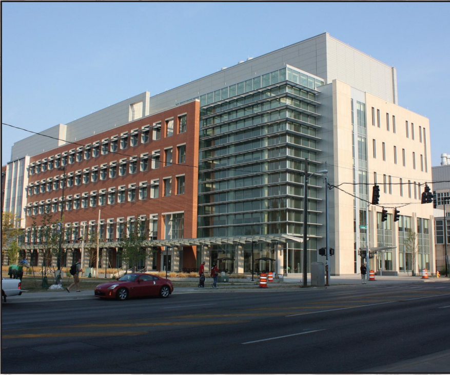
The Biological Pharmaceutical Complex, dedicated in January, is located on South Limestone and is home to the College of Pharmacy. It includes a five-story atrium, two 219-seat auditoriums, a 110-seat classroom, a 54-seat classroom, a teaching laboratory with compounding laboratory and patient assessment rooms, and nine group-learning rooms.
