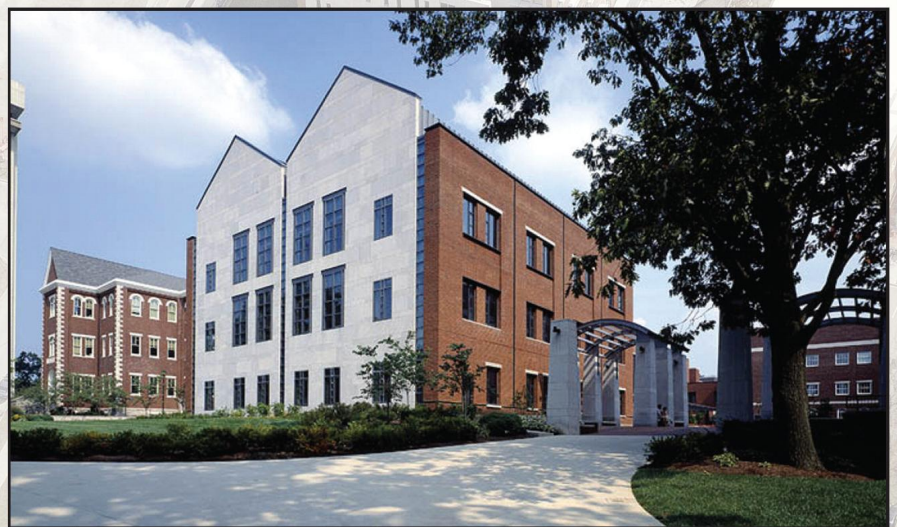
Old With The New: The Ralph G. Anderson Building, right, completed in 2002, uses the same materials (limestone and brick) as the adjacent Miller Hall (1898) but reverses them.
