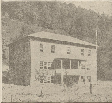
SCHOOL AND ADMINISTRATION BUILDING, KINGDOM COME.
