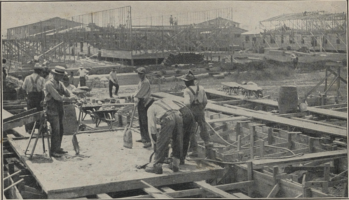
Constructing Camp Zachary Taylor at Louisville, Ky.
