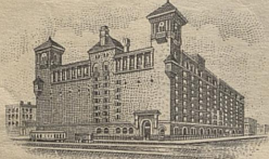
52ND STREET BUILDING
