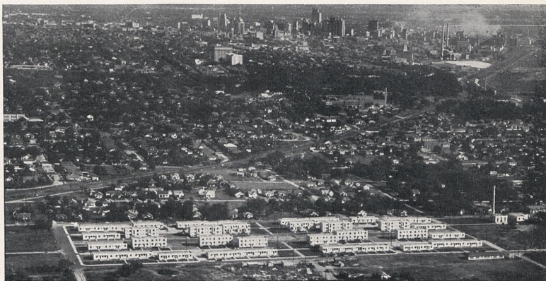
Cedar Springs Place, PWA Housing Division project in Dallas, Tex., opened in 1937.
