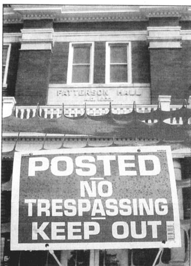
Patterson Hall, a residence hall on North Campus, is closed for renovations this semester.
