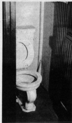
A paneled portion of the kitchen forms this "water closet" for student apartment near campus. The shower stall is a similarly paneled-off portion of the kitchen.
