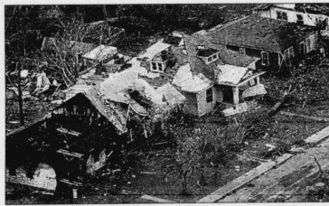
A house was destroyed by recent storms in eastern Tennessee.
