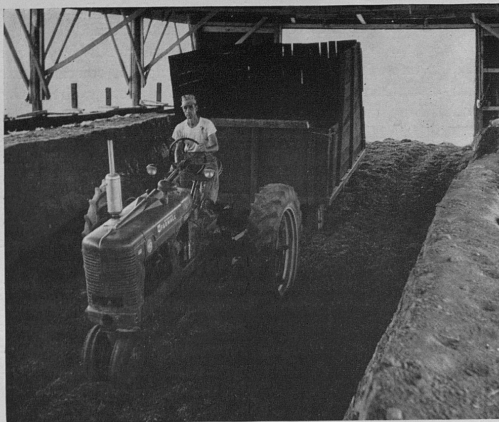
Fig. 4.— This trench silo is in a shed attached to a livestock barn. It provides low-cost and safe storage for grass silage.
