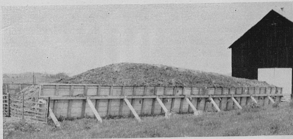
Fig. 2.— A concrete-stave bunker-type silo on the University of Kentucky Mercer Farm. This silo requires no upkeep and is well suited to self-feeding operation. Bunker silos cost less to construct than upright silos. However, more spoilage of silage occurs in bunker silos.
