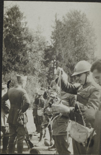
GAS MASK INSPECTION
