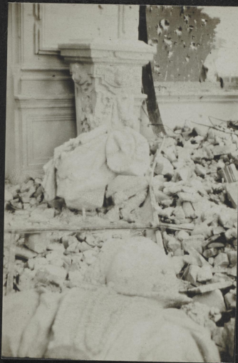
FALLEN STATUES IN MAIN HALL
