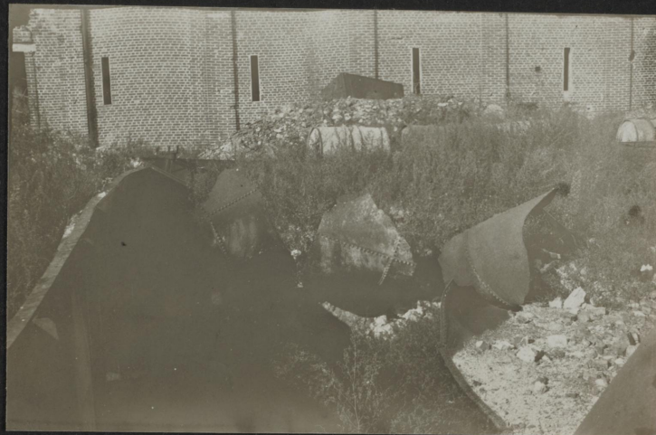
3/4 " PLATE STEEL TANK TORN BY SHELL
