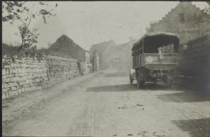
"DUSTY ROAD" NEAR BOUCY-LE-LONG.
