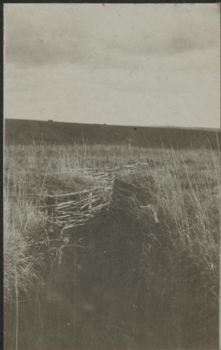
RESERVE TRENCHES ON HILL ABOVE CHAVIGNY
