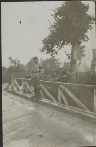
GUARD ON BRIDGE AT PONT-ARCY
