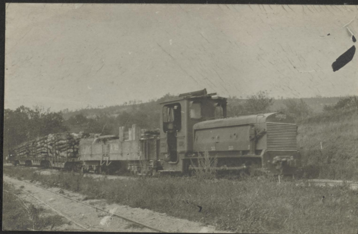
GASLINE ENGINE HAULING TRENCH TIMBER - ALONG AISNE RIVER NEAR VAILLY.
