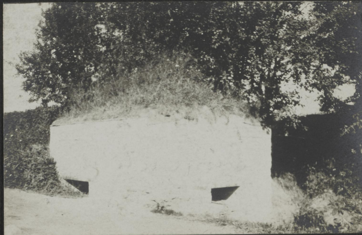
GERMAN "PILL BOX" SOLID CONCRETE MACHINE GUN HOUSE
