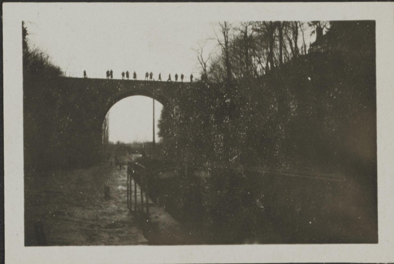
BRIDGE OVER CANAL
