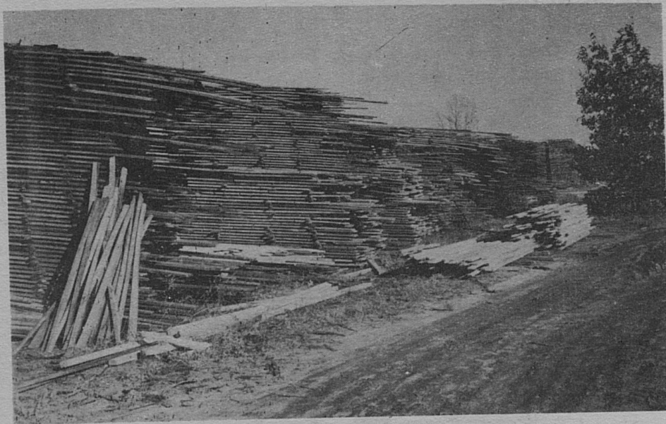
Fig. 6. - Excessive Overhang of Boards in Rear of Piles. Note also the poor foundations.
