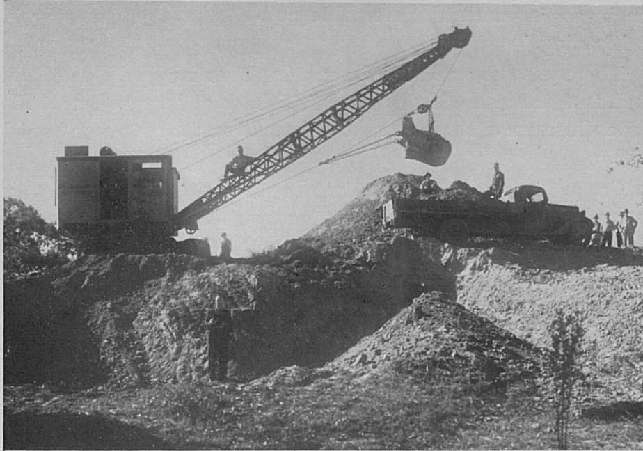
Trucks and drag line used by Henderson County farmers to handle marl.
