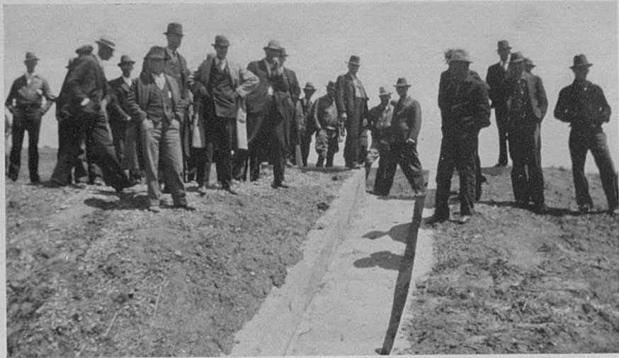
Concrete flume for lowering water from a terrace to the outlet.
