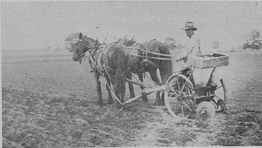
Fig. 3. A "One-Man" or "Picker" Potato Planter.
