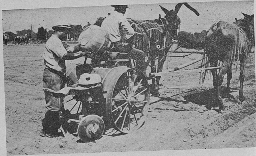
Fig. 2. A "Two-Man" Potato Planter.
