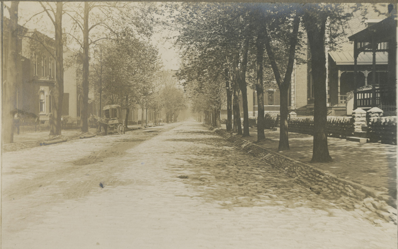
Overton Street looking North from 6th Street 3-11-10
