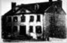
THE HOUSE BUILT BY THE FIRST SETTLERS OF THE TOWN
