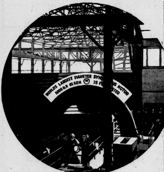
This 5,000 h. p. motor in the Columbia Steel Company's plant, with its frame of arc-welded steel, is physically the largest synchronous motor ever built.
