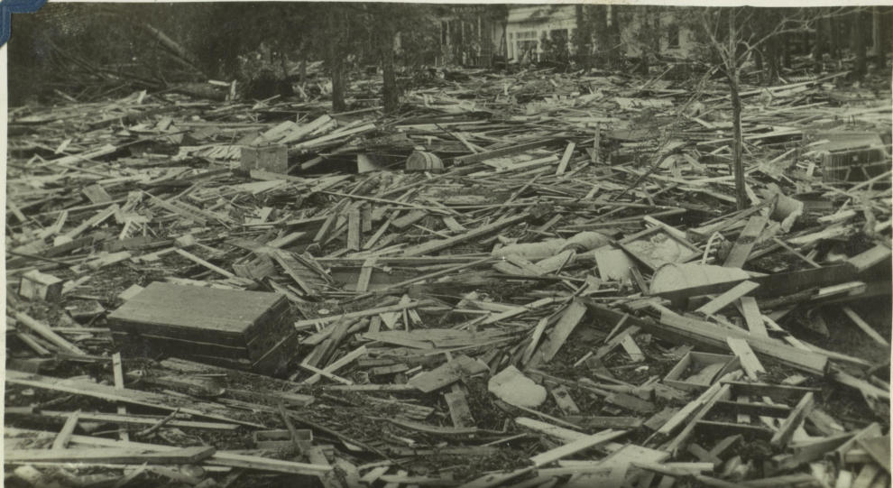
350 homes wrecked, 1100 damaged. 12 lives lost. 100 injured in Hancock Co. Hurricane Sept. 19, 1947.
