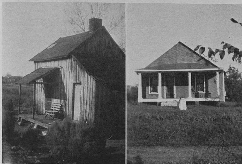
Before and After: The home demonstration agent in Christian county furnished plans and the colored family living in the house did all the work of remodeling.
