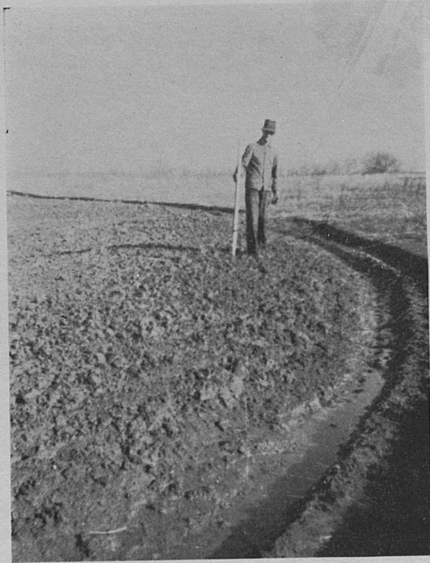
A McCracken county farmer shows terraces he made with a farm tractor, on lines laid out by the assistant county agent.
