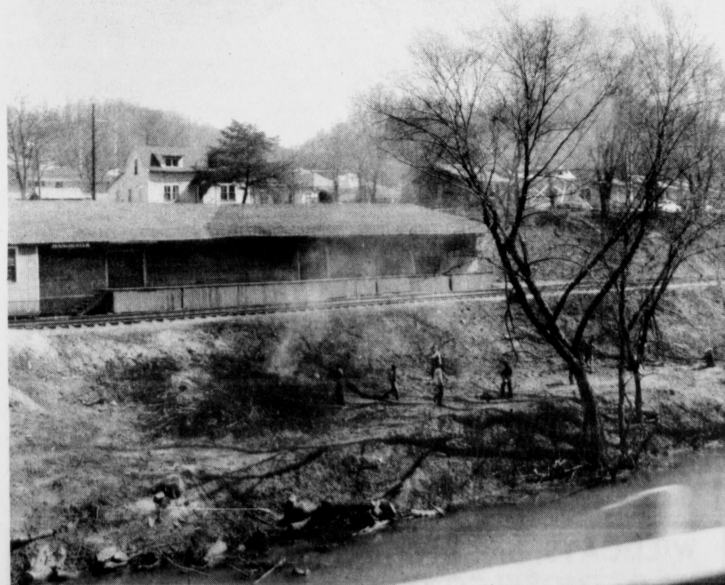
"Happy Pappies" clear off a creek bank in Manchester to aid water drainage. The men work under the Welfare, Education and Training Program
