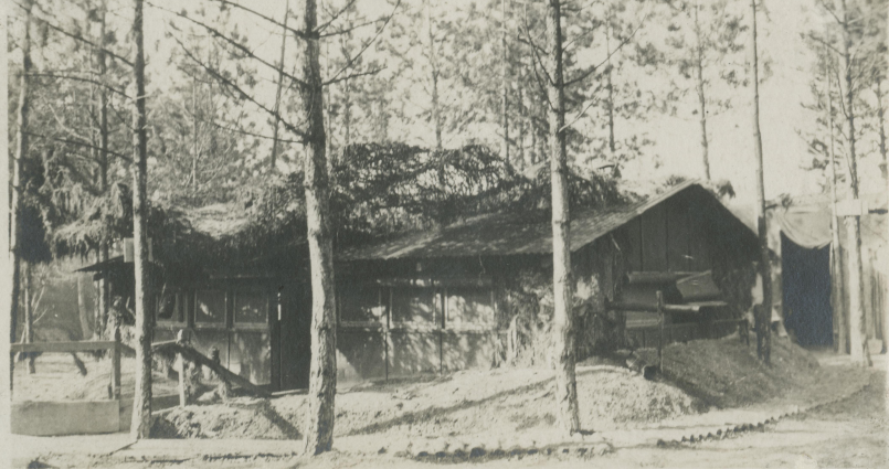
Kitchen & Dining room at LaPlaine, France. 662.
