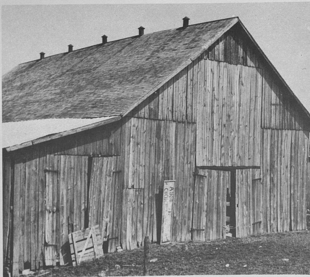
Fig. 28. — You have little control over curing conditions in a barn such as this. Sheds placed on the sides of a burley barn cut off ventilation completely. Also, ridge ventilators are useless.
